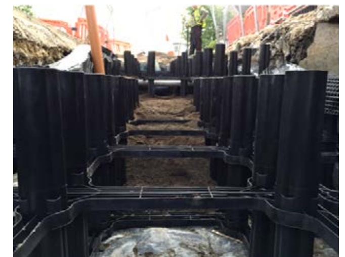
'Box-crate' Tree-planting as a Storage, Water-cycling and Attenuation SuDS Component (images courtesy: DeepRoot UK)
